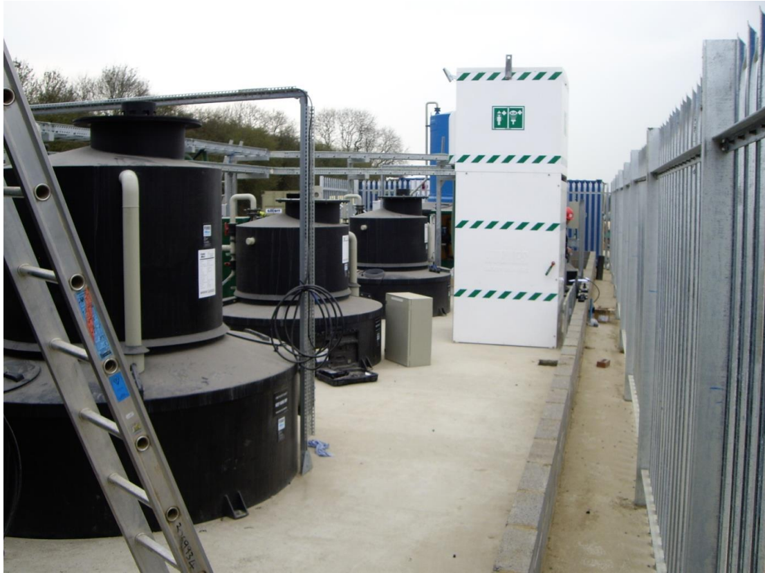
Bunded chemical storage tanks & Dosing pumps being installed at Milton Keynes.
