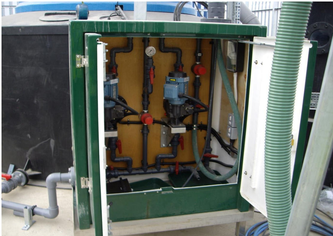
Bunded chemical storage tanks & Dosing pumps being installed at Milton Keynes.
